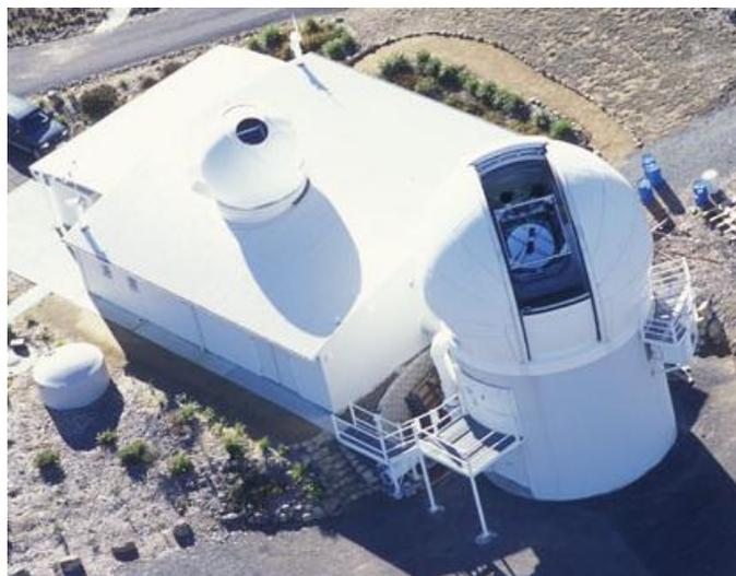
Fig 1: 1.8m telescope with co-rotating observing floor
